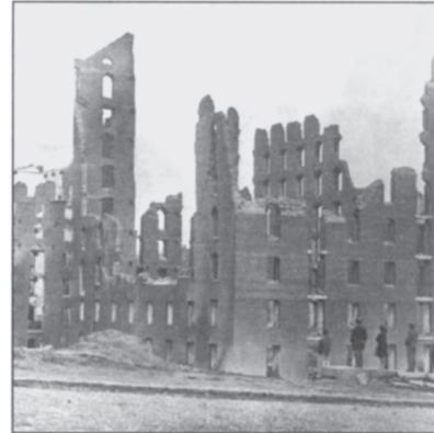
Ruins of the Gallego Flour Mill in Richmond, Virginia, immediately after the Civil War.
