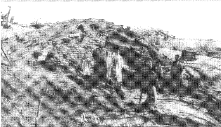
A family stands in front of their sod dugout home in Kansas. Such dugouts were usually temporary until a more permanent “soddy” could be built.
